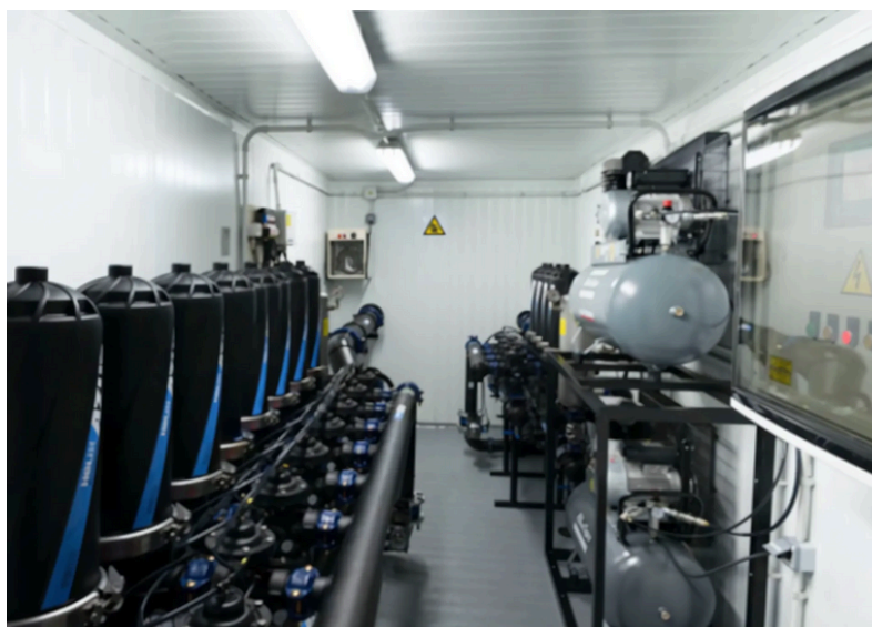
Side stream filtration in the cooling tower of thermal power plant.
